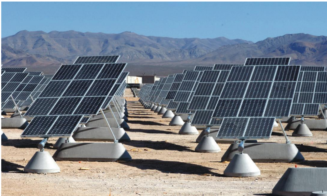
Figure 3. One-axis tracking solar power plant
